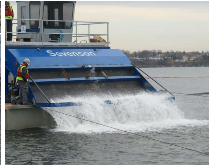
Spreading Sand Over Sediments
